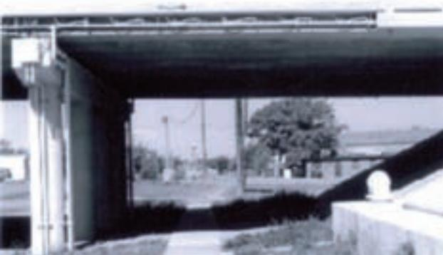
A well known and well documented geothermal installation is the SERSO pilot plant in central Switzerland, which went into operation in 1994 and is still running. Aim of the installation was to prevent ice-formation on a highway bridge surface.
